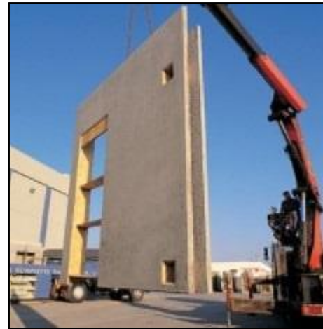
Fig : 14.6 : Precast Flat Panel System
