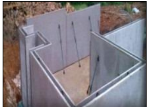
Fig : 14.10 : Twin Wall Technology
