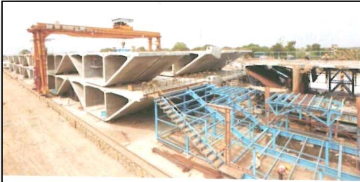
Fig :5.9: Casting Molds With Staking Yard For Segment
